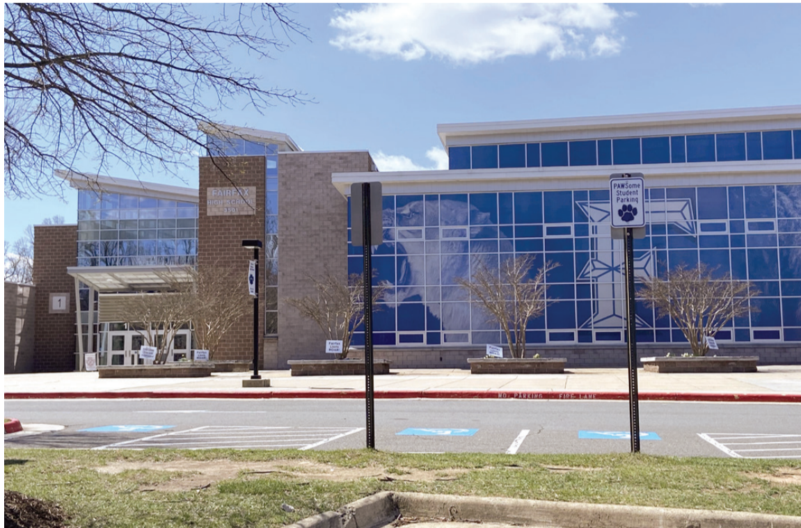
Fairfax High School off Blenheim Boulevard.
